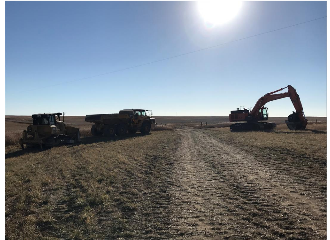
Photo of Drilling Lease Construction in Gensource' Vanguard Area
